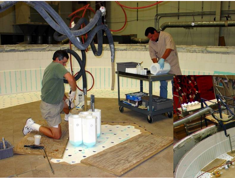
Machine and install 1681 ceramic fiber boxes in silicon carbide tub.
