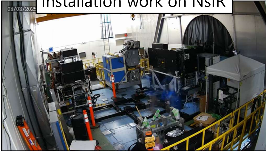
Installation work on NsIR
