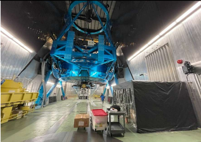
Alignment work on Obs floor
